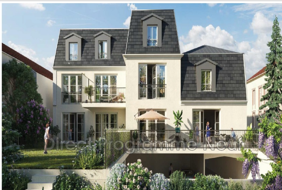
Apartment ref. 802N6972A Suresnes
